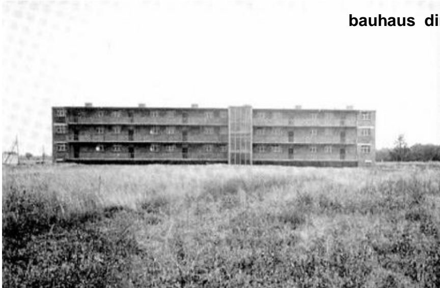
residential complex Dessau - Törten 1930
